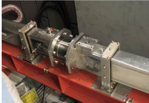
Figure 7. A photo of the same part shown in Fig. 5 taken from the opposite side after the refurbishment. One can see that designs of support frames and a bellows have been changed.
