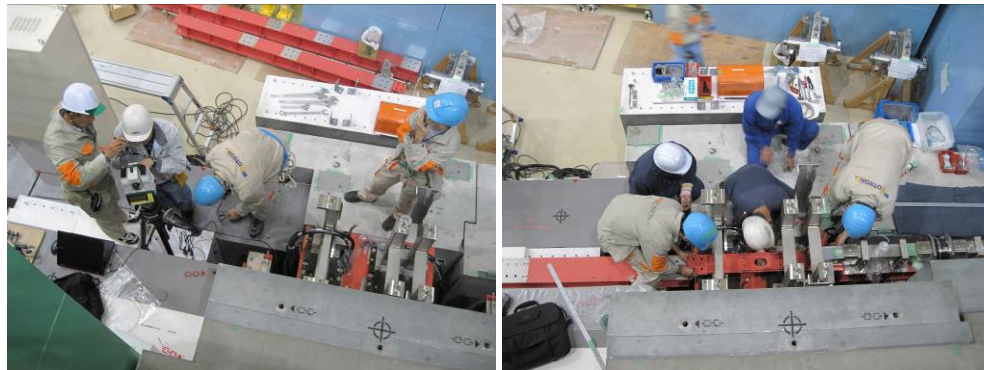
Figure 6. Re-alignment work at AMATERAS.
